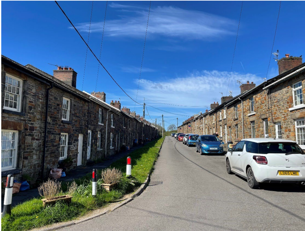
Plate 166: Looking west from the east end of Park Terrace (April 2024)
