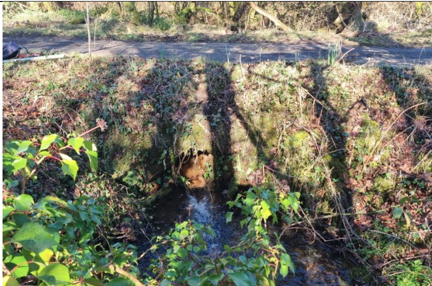
Photo 4: A view of the downstream culvert outlet, looking upstream.
