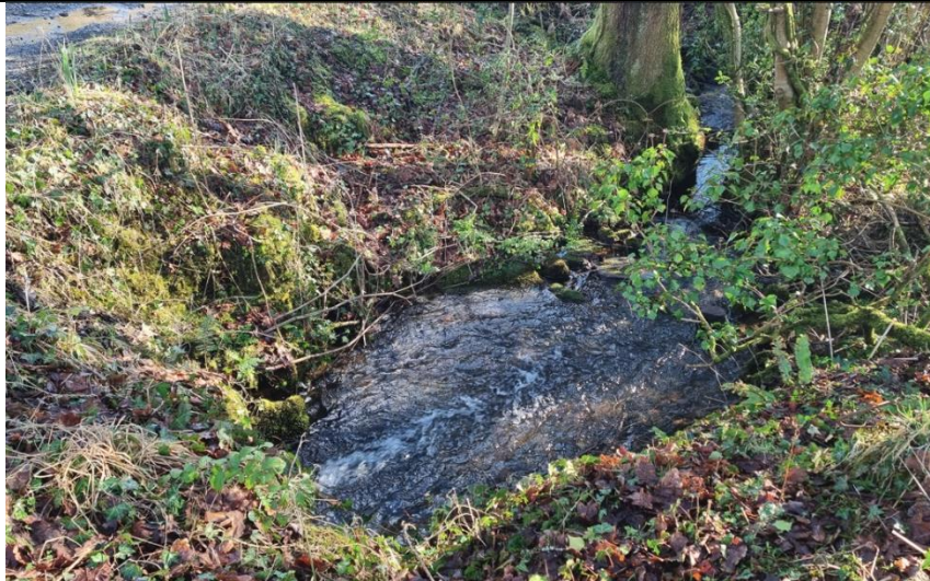
Photo 3: A downstream view from the culvert outlet.
