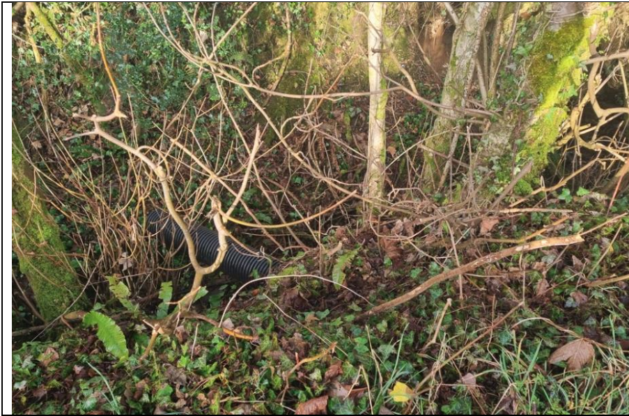
Photo 3: Pipe outfall assumed to be land drainage from the field to the east of Cwm Risca Lane.
