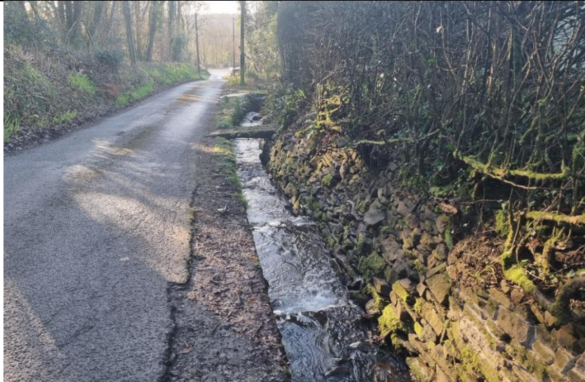
Photo 3: A view of the downstream extent of the watercourse from the location of the outlet.
