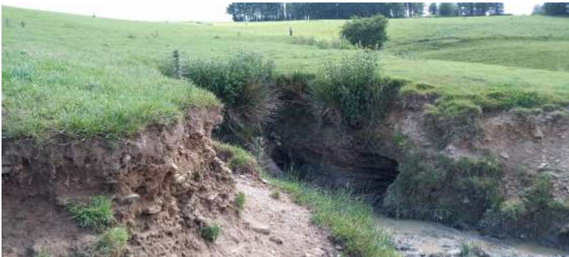
Photo 5 Example of ground conditions on site.
